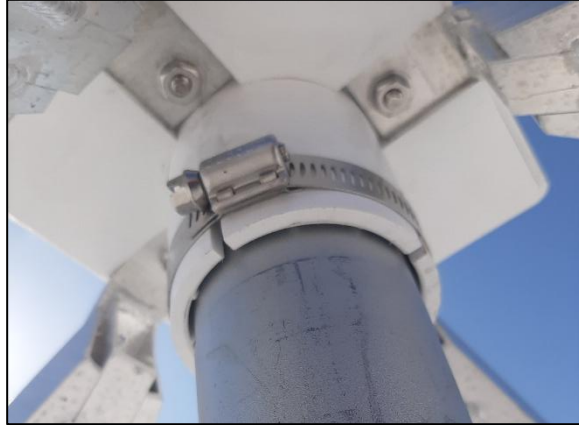
Figure 9: Electronics unit screw clamp
