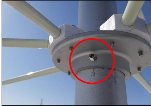
Figure 7: Location of one set screw on element support plate
