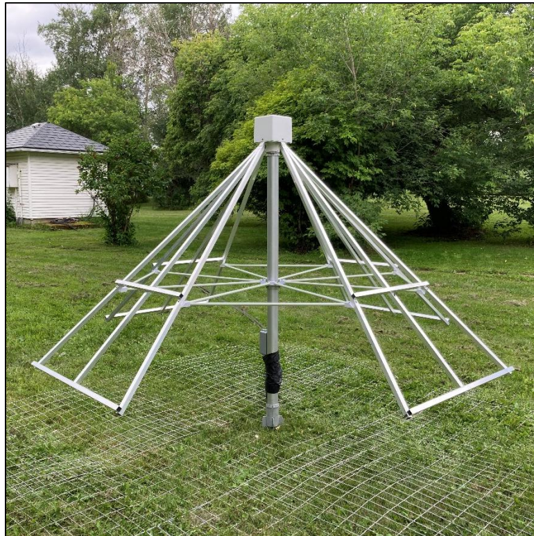
Figure 6: Finished antenna installation with ground plane
