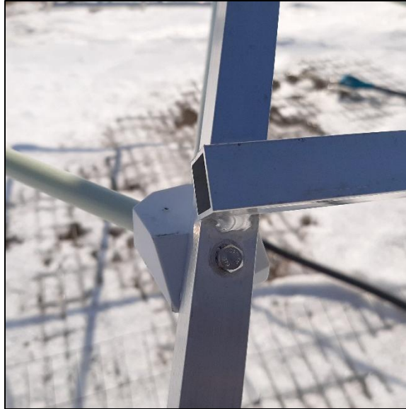
Figure 19: Element to element support connection
