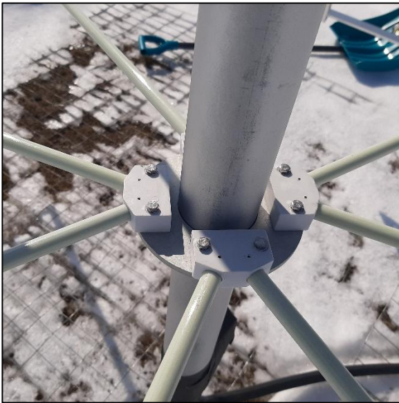
Figure 14: Element support plate with element supports
